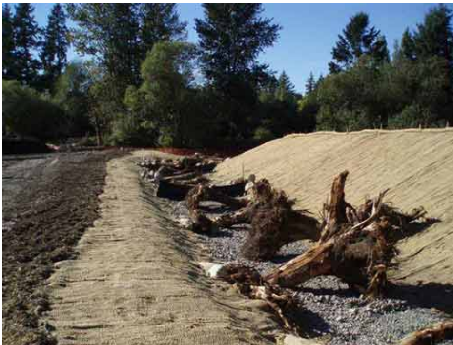
LWM placed as tow protection during channel reconstruction
