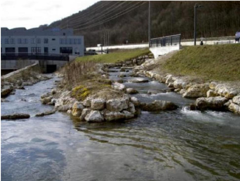
*By-pass fish passage at culvert*
