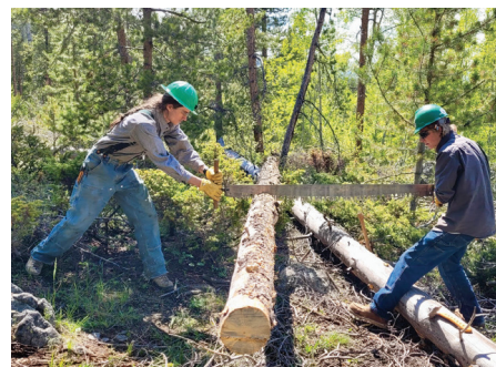
Wilderness areas do not allow mechanized tools and equipment, so HTA staff receive training and federal saw certifications to remove hazard and fallen trees in Grand County's five wilderness areas. Photo by HTA.
