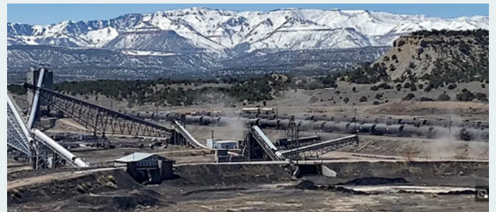
Pictured above: the Wildcat Loadout Facility near Price, Utah, courtesy John Weisheit and Aspen Journalism.
