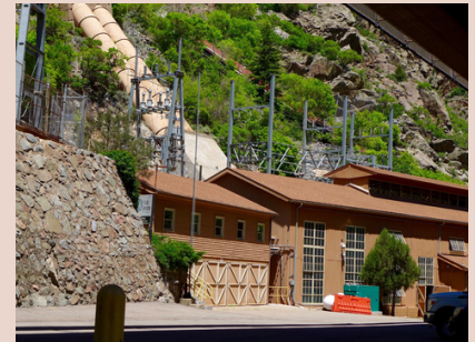
Pictured above: Located in Glenwood Canyon, the Shoshone Generating Station is more than 100 years old, and is the cornerstone for water rights in the Upper Colorado River.
