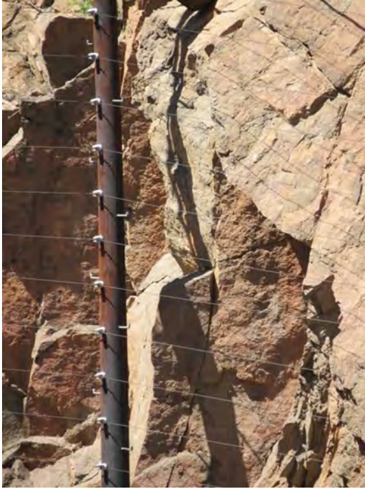
Figure 3-18 Close-up of Rockfall Alarm Fence in Byers Canyon
