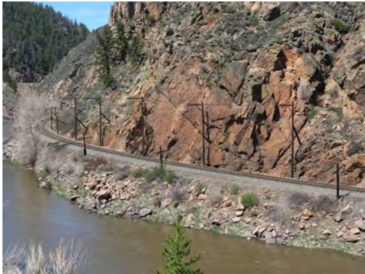
Figure 3-17 Rockfall Alarm Fence in Byers Canyon
