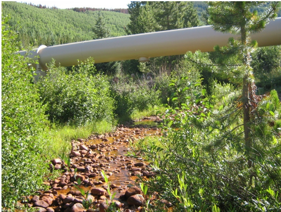
Jim Creek at the Fraser River canal pipeline
