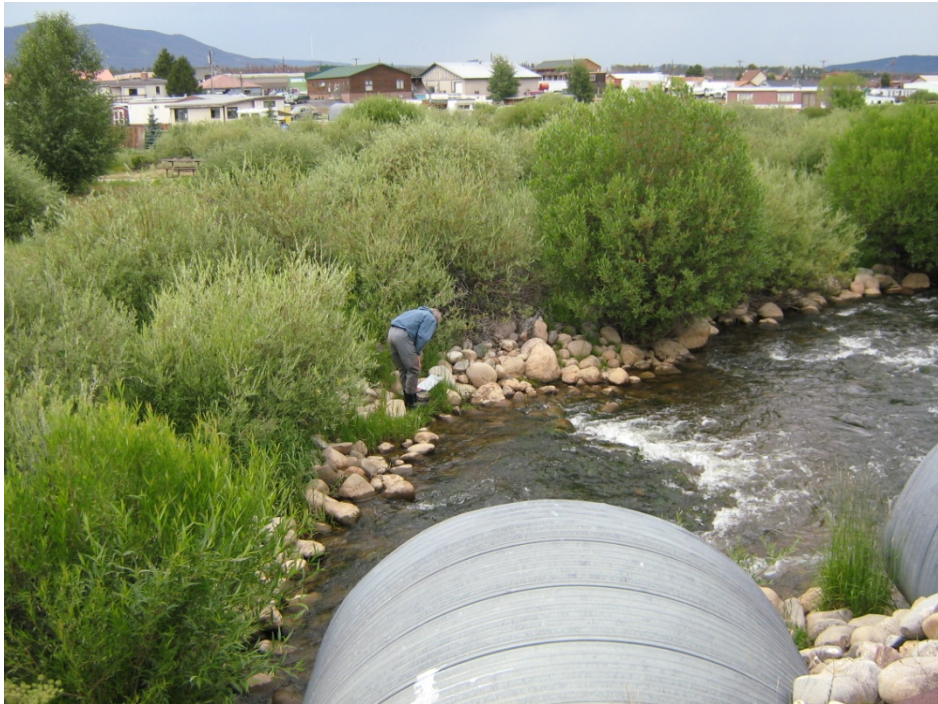
Fraser River Culverts at South Wapiti Drive
