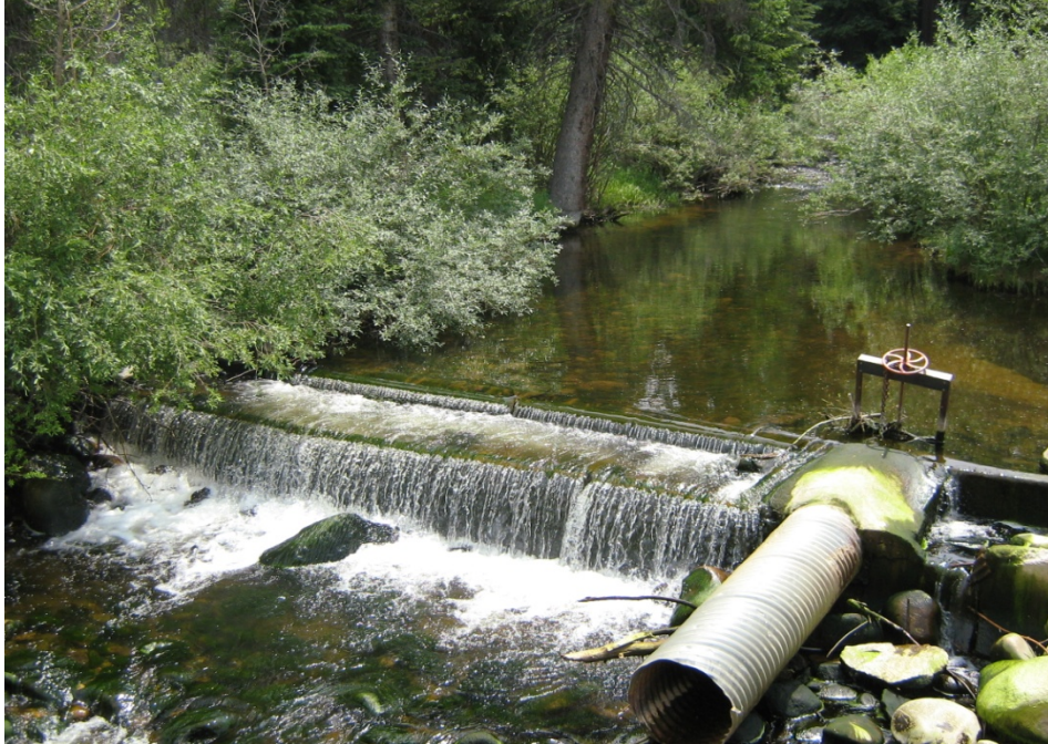
Vasquez at private diversion structure in the town of Winter Park
