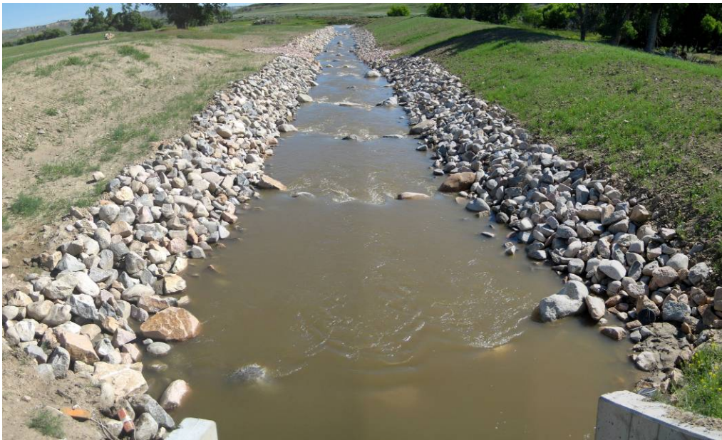
Fish by-pass channel (stepped)
