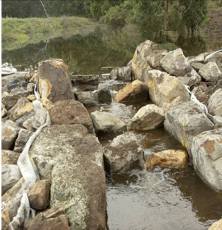
Low flow stepped boulder fish passage structure
