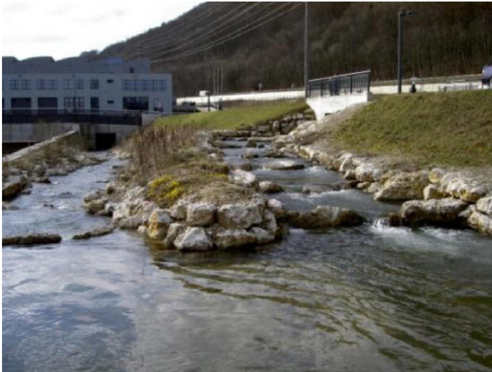
By-pass fish passage at culvert
