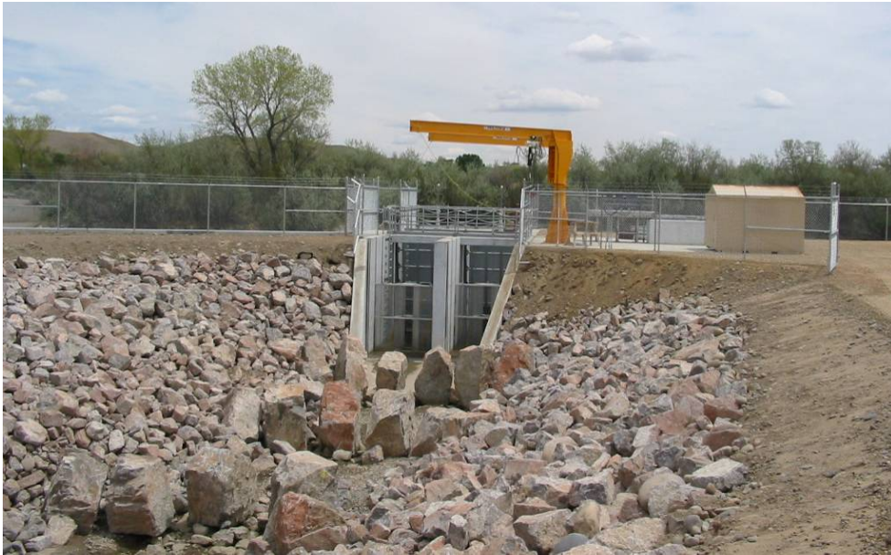
Fish passage structure with sorting facility (under construction)
