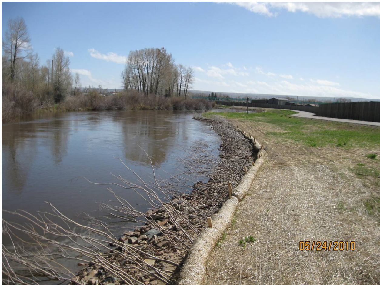
Stone toe protection with willow stakes and coir (immediately following construction).
