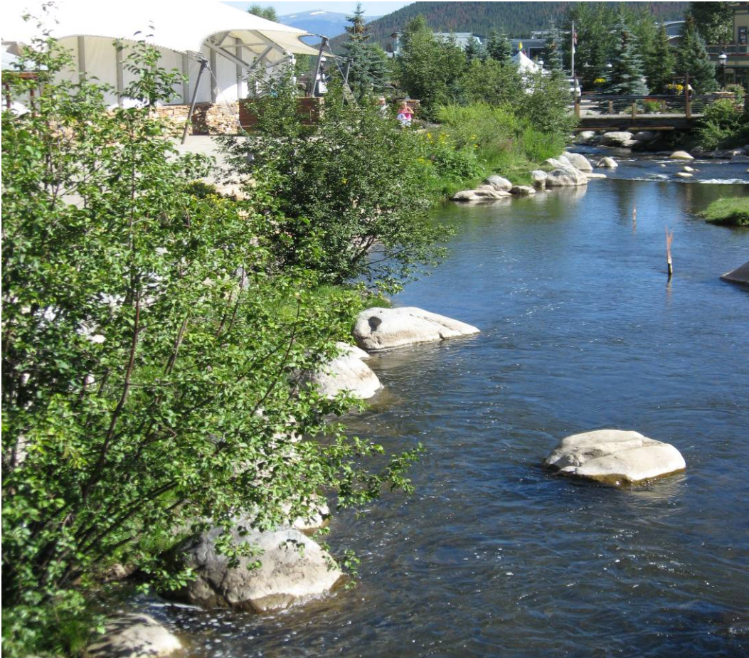
Stone toe protection with well established planting bench
