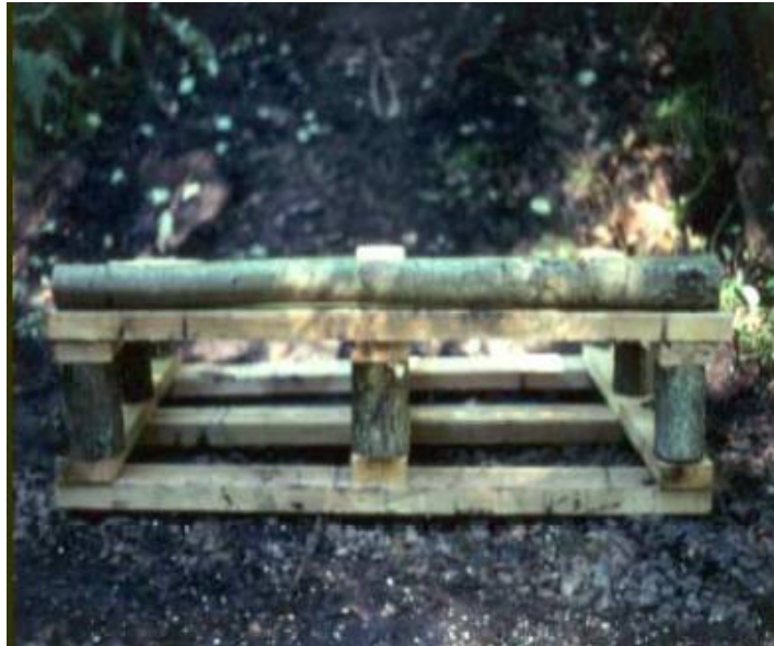
Photo 1. Fabricated Lunker Ready for Installation
