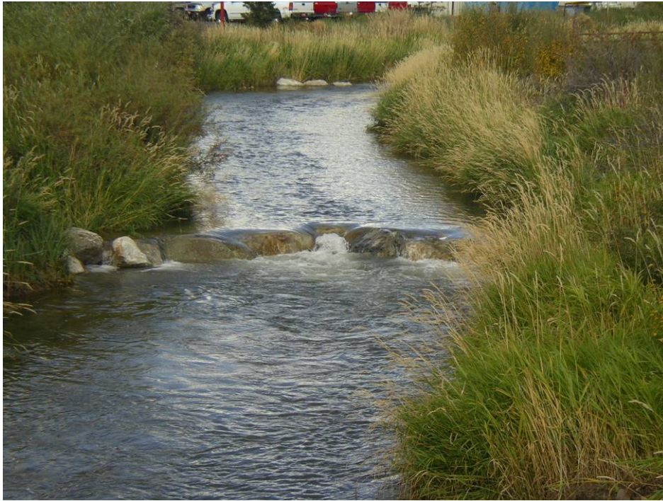
Boulder cross vane for bank protection and grade control.
