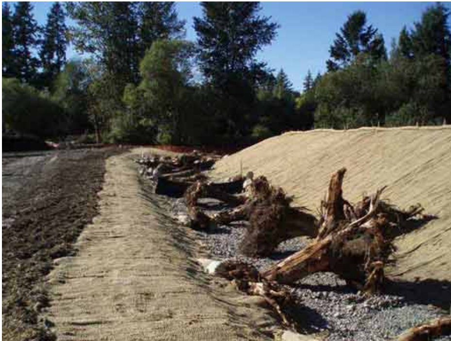
LWM placed as tow protection during channel reconstruction
