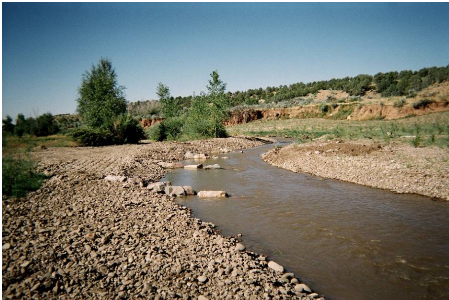
J-weirs in series along right bank during channel reconstruction
