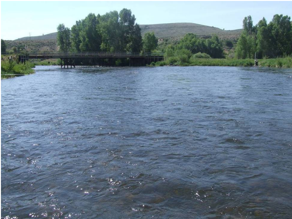
Photo 1. Looking upstream towards bridge (03Jul07)
