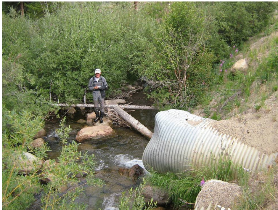
Photo 1. Downstream of RC1 PHABSIM Site at culvert under County Road 8
